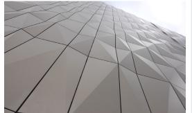
This project involved a refurbishment of the exterior façade of the Marriott Hotel, Portsmouth, including the installation of new glazing and cladding systems, designed to bring both aesthetic and building efficiency improvements.
